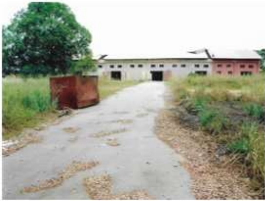
Plate 5: Burglarized Government Warehouse at Ekorinim
