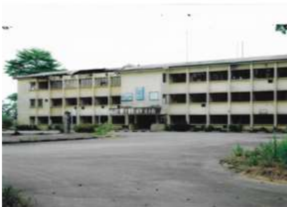
Plate 3: State Ministry of Works Building at Ekorinim
